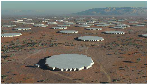
Figure 3: SKA dense aperture array station made up of 3 m x 3 m “tiles” for about 500 MHz–1 GHz. Graphics: Swinburne Astronomy Productions and SPO.
