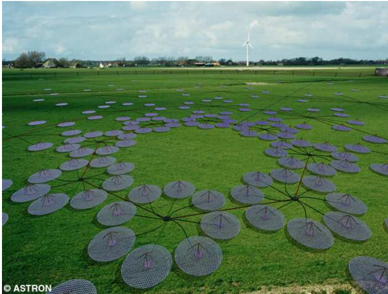
Figure 5: Model of a LOFAR station with low-frequency antennas (by courtesy of ASTRON).
