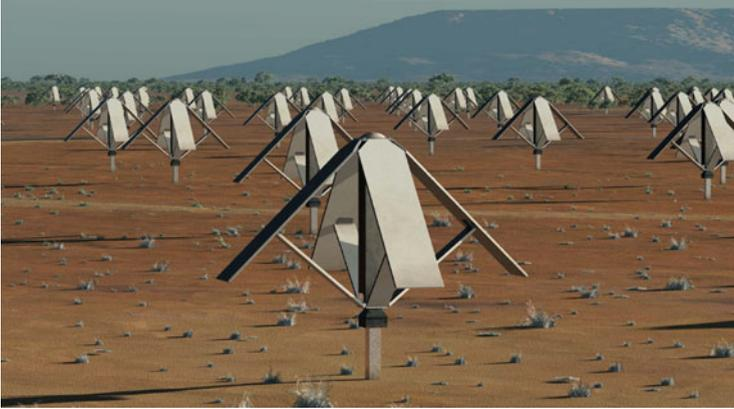
**Fig. 1.6** SKA sparse aperture array station of dipole elements for low frequencies of about 50–350 MHz. Graphics: Swinburne Astronomy Productions and SKA Project Office (SPO)
