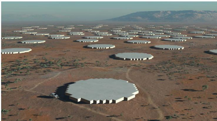
**Fig. 1.8** SKA dense aperture array station made up of 3 m x 3 m “tiles” for medium frequencies of about 500 MHz–1 GHz. Graphics: Swinburne Astronomy Productions and SPO
