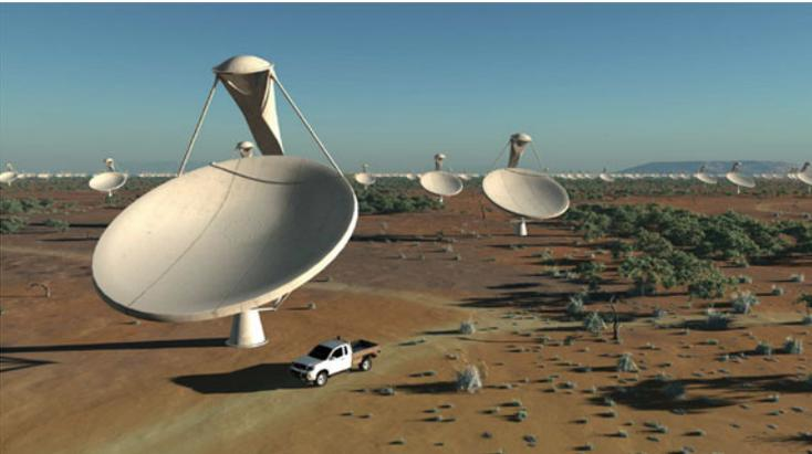
**Fig. 1.7** SKA parabolic dishes for medium frequencies of about 350 MHz–14 GHz. Graphics: Swinburne Astronomy Productions and SPO
