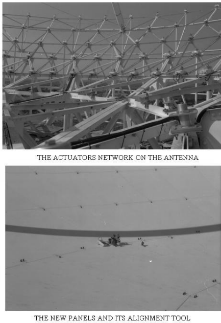
Fig. 6. Installing the aligning the system
