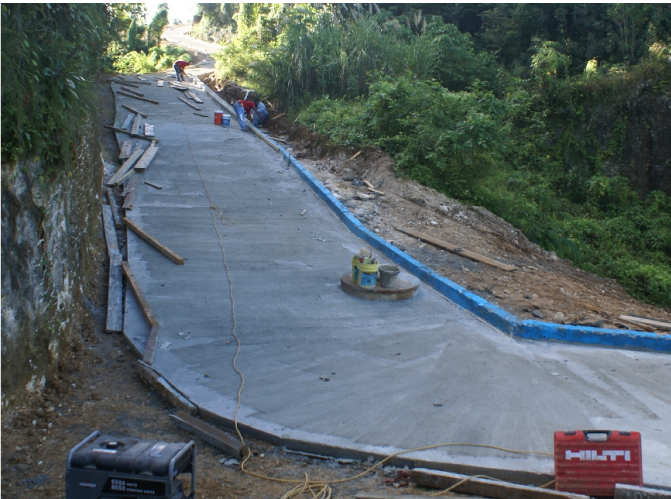
Access Road (then nearing completion)
