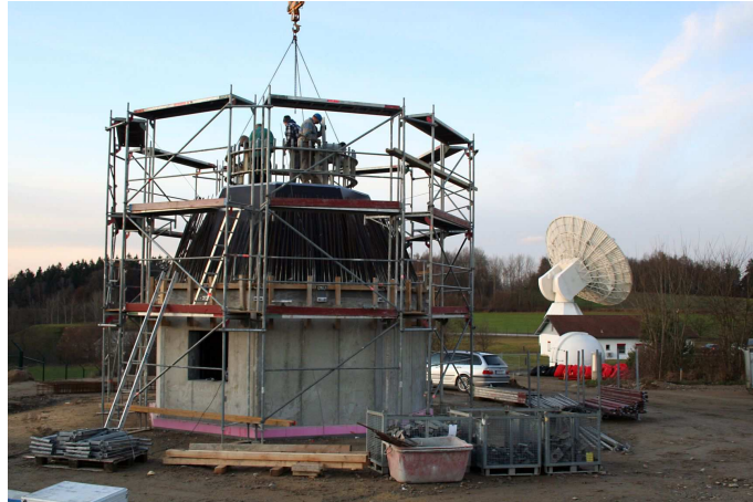
Figure 3. Construction of the concrete tower
