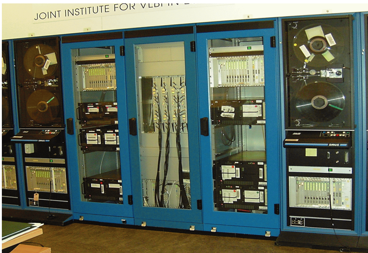
Figure 4: Mark5 Installation at JIVE
