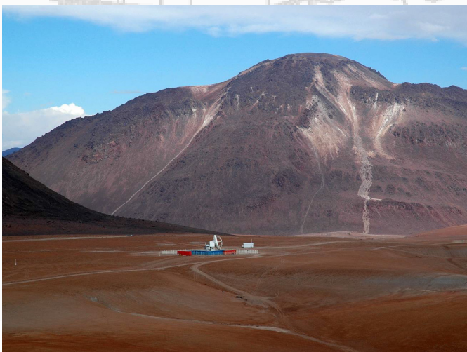
The APEX telescope site seen from one of the nearby hills. The containers are in front of the telescope and the white power house containing the generators can be seen to the right.
