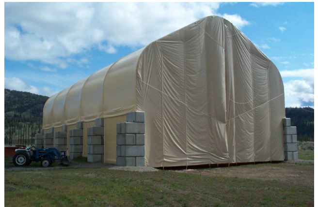
The upgraded hangar. An extra 20-ft section and the curtain-style door were added in Fall 2002.
