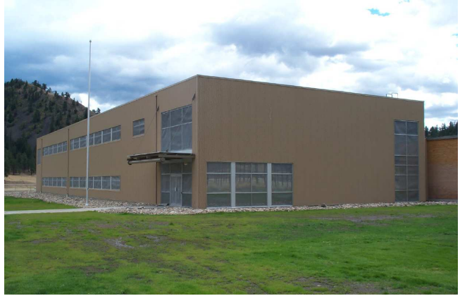
An exterior view of the new building. Note the wire mesh over the windows, to help reduce interference radiated from within.
